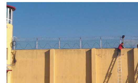
Figure 3. Perimeter Monitoring Site of a Prison in Harbin
