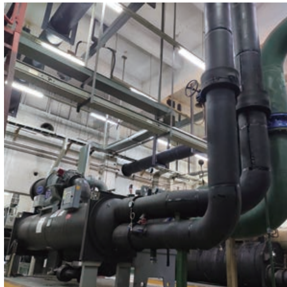
Refrigeration station pipeline renovation
