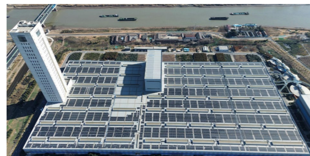
Distributed PV power generation project of YOFC Marine
