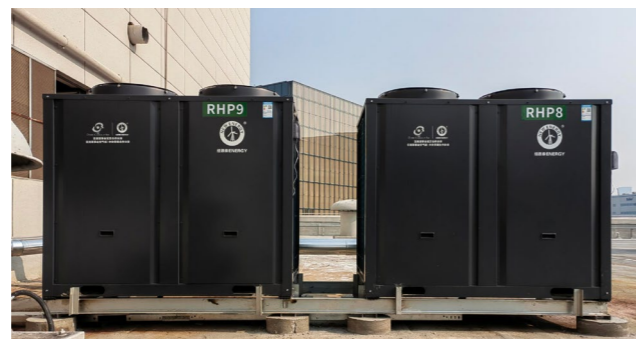
Upgrade project of replacing steam with air-source heat pumps
